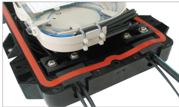
Drop Cable Installation
